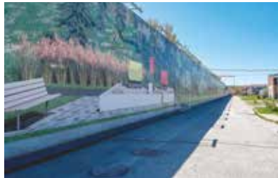
TEMPORARY NOISE SCREEN installed along Champlain Avenue to limit possible noise from operations.
