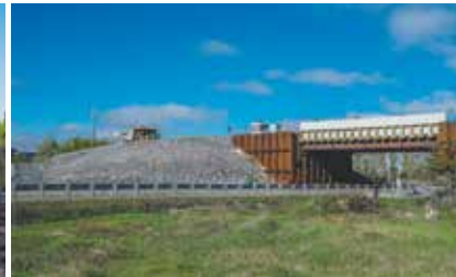
TEMPORARY BRIDGE BUILT OVER HIGHWAY 117, to limit traffic disturbances on the highway during work.
