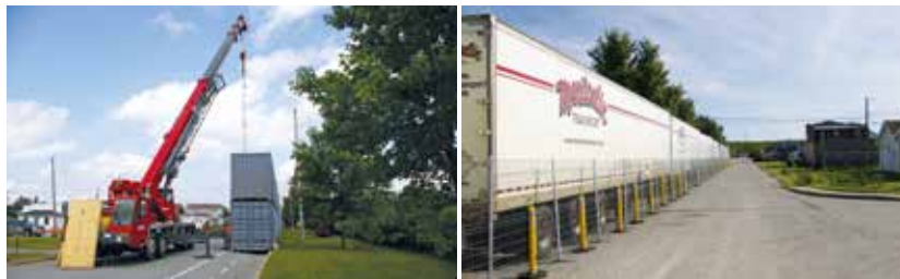
DURING TEMPORARY NOISE SCREEN INSTALLATION
