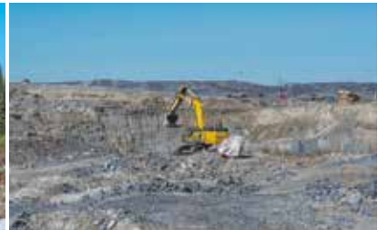
PIT SURFACE STRIPPING AND EXTENSION
